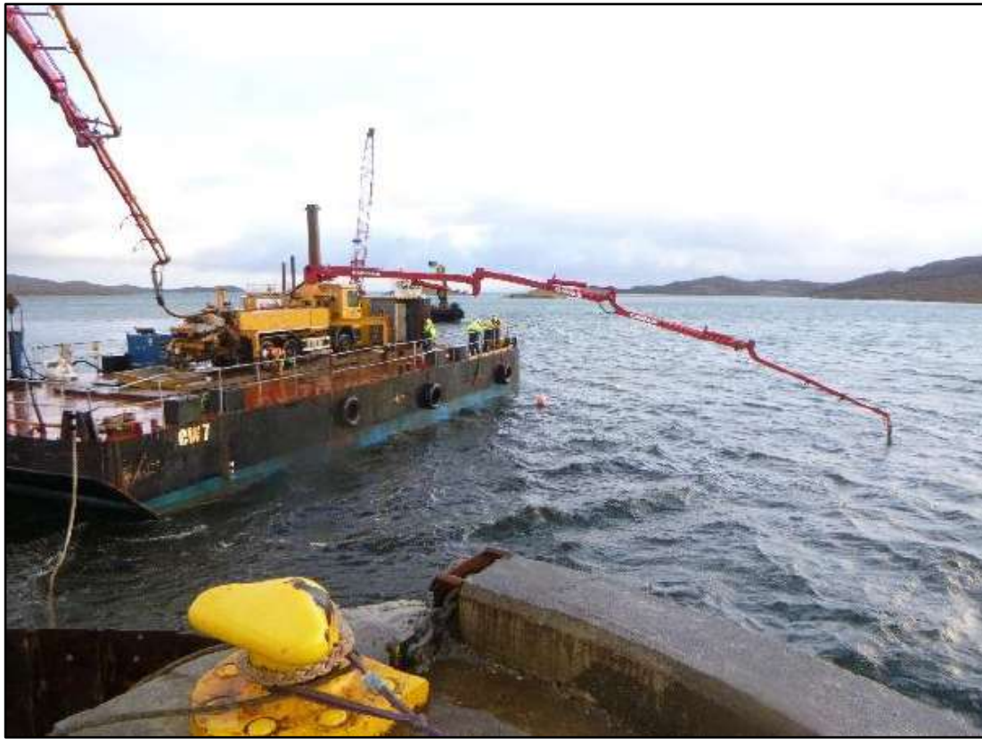
Underwater Placing of Caisson Concrete Foundations (Photo - Wallace Stone LLP)
