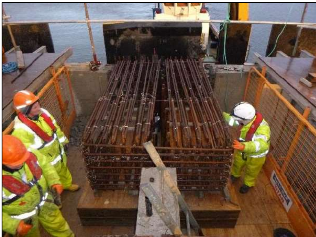
Installation of Reinforcing to Pier Bollard Foundation (Photo – Wallace Stone LLP)
